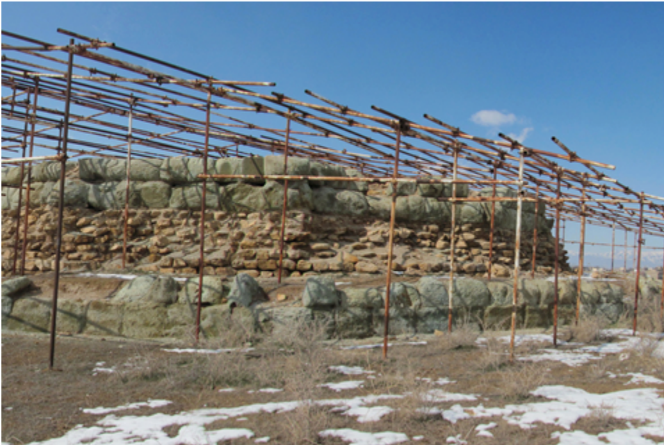
The three platforms of the structure. The first and the third layers are built in cut stone and are dodecagonal in form, while the second structure is circular.
